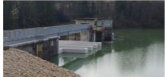
Upstream view of the PKW
